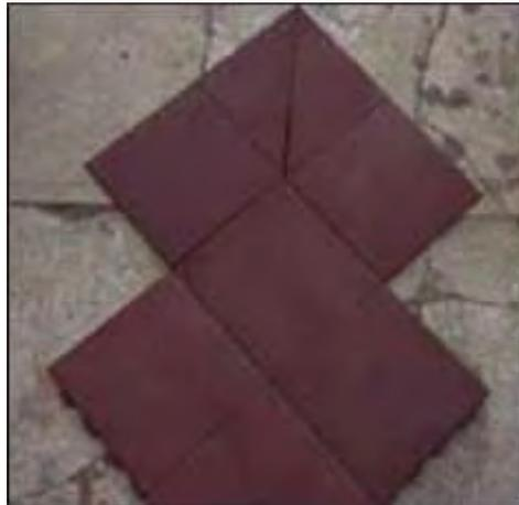
**Factory edges:** Always butt **factory** edge to **factor** edge. Cuts go against the wall or other vertical surface. You can make your own "factory edge" in scraps by using a carpenters' square to square the piece and undercutting. Keep in mind, when installing the half (1/2) tile-mat-block for the "step & repeat" pattern, the cut edge will not be against the factory edge only at the very end of the surfacing and flooring being installed.
