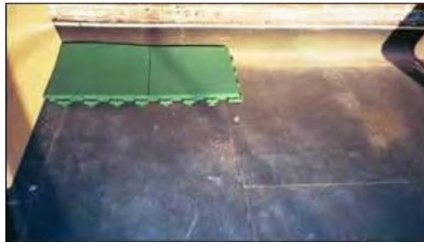
Place the next piece in by dropping the female interlocks of the second product directly over the male interlocks of the first product as seen below. As a result the interlocks from product-to-product will be completely covered and interlocked. Product orientation to these products and all of the following products must be identical to that of all odd numbered rows.
