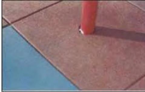
You can establish the field without installing the piece that will eventually have to be cut, by using full-length scraps as spacers. Once the row has been established, complete the area around the obstruction. If the slope around the drain or object is so great as to keep the products off the adhesive ...sandbag the area overnight. Below is what the final installation should like when completed.
