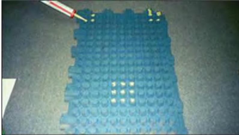
Most installations will be with a one part adhesive. This adhesive comes in a large tube, so a larger corking gun is needed for gluing applications. For solid sub-surfaces, be sure to glue the outside perimeter cones, (feet, legs) of the products located underneath with a small application in the middle. After setting it in place, begin gluing the male interlocks of that product which should be located at the 3 and 6 o'clock positions.
